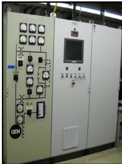
New System Installed On-Site
